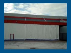
Heavy Duty Curtains suspended from overhead track
