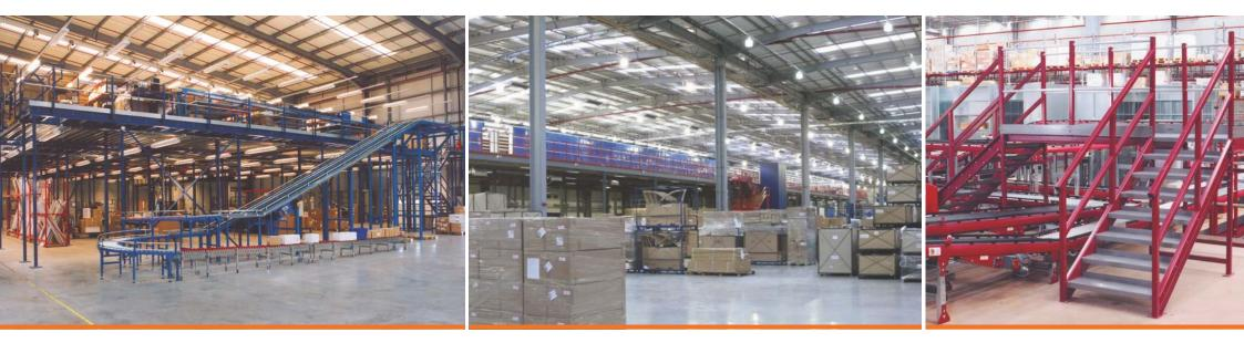
A mezzanine floor offers additional work or storage space without adding to the building footprint. Mezzanine floors are supported floors erected within a building independent to the structure that allows you to take full advantage of the vertical space to expand your business in a cost effective way.
