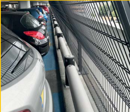
iFlex Single Traffic High Level guarding boundaries in a multi-storey car park.
