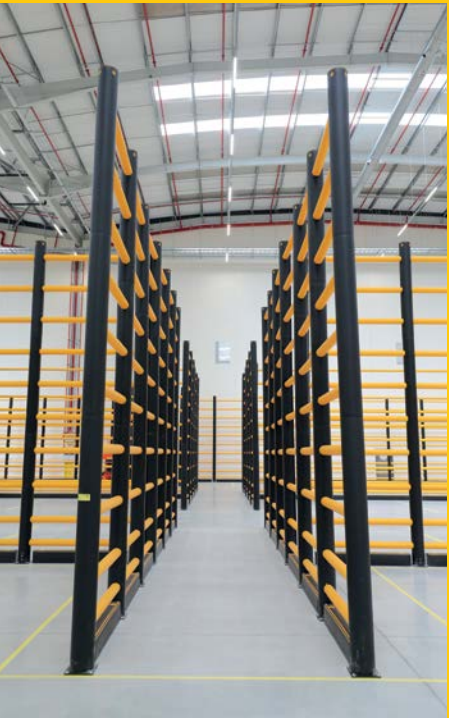
iFlex Topple Barrier providing a safe route between storage bays.
