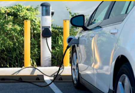
Bollards protecting electric car charging point.
